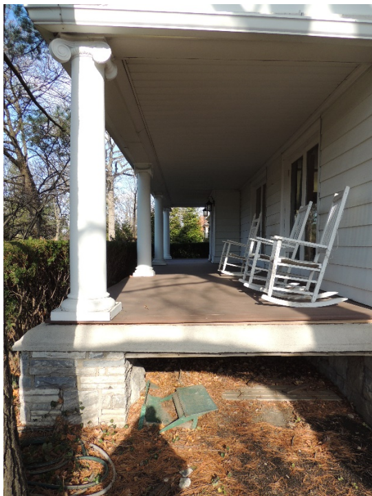
4. Bagley House-Front Porch Showing marble columns and marble facing on supports
