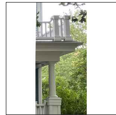
EXISTING FLAT ROOF CORNICE
