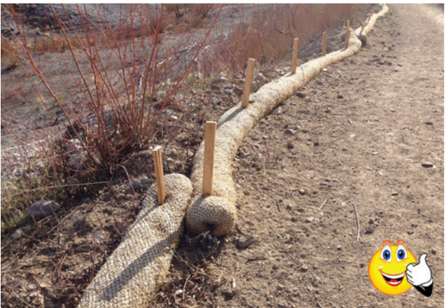
Good fiber roll installation Great overlap of fiber rolls - gaps between sections of fiber rolls often allow runoff to concentrate, which can result in accelerated erosion.
