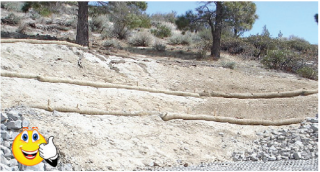
Good slope erosion protection with overlapped ends of fiber rolls.
