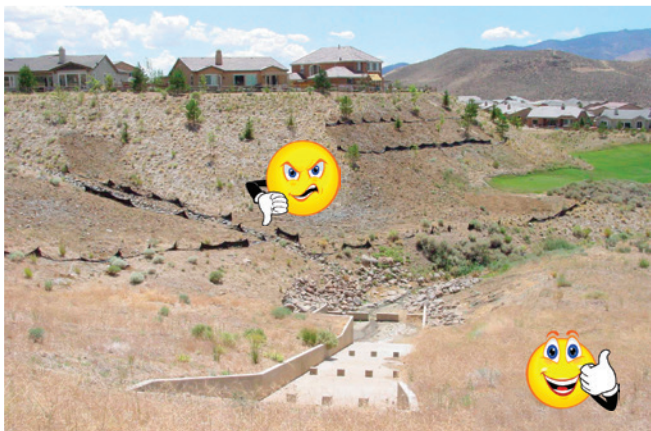
Large storm drain outlets may require concrete structures for conveyance, velocity dissipation and erosion control designed by registered civil engineers. The slopes in this photo appear to be stabilized. Now it's time to remove silt fence and stabilize the keyed trench.
