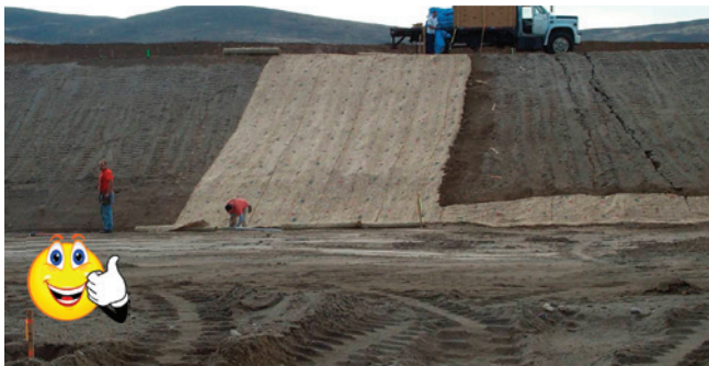
Good application of erosion control blankets to stabilize highly erodible soils on new cut slopes at this construction site.
