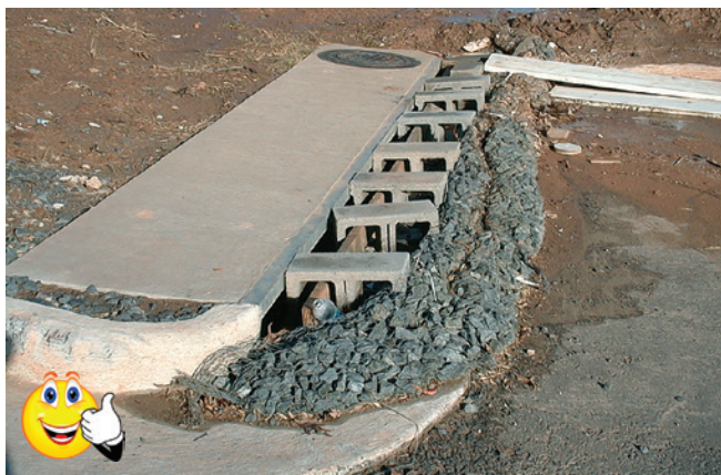
Excellent use of concrete blocks and rock in mesh bags to protect a large storm drain inlet located within a large construction site. Note the 2" x 4" board through the concrete blocks for reinforcement.
