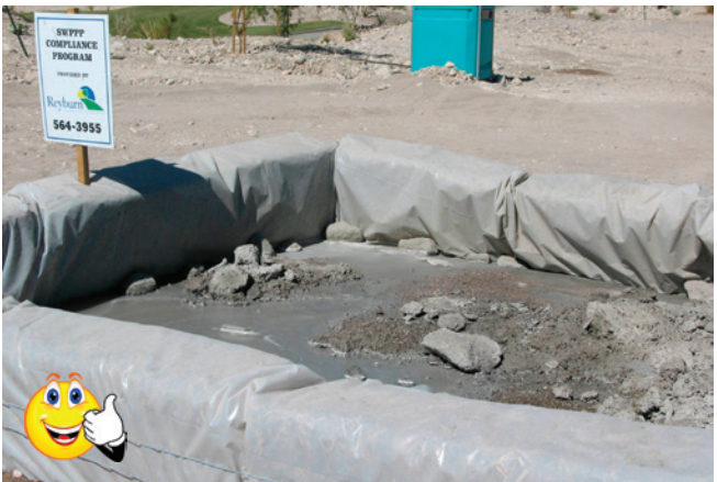
Wash concrete delivery truck chutes and equipment in dedicated concrete washout areas. Straw bales covered in plastic sheeting or plastic kiddie pools may be used. This area must be labelled in the SWPPP maps and marked with signage on-site.
