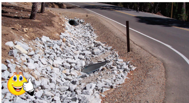
Excellent rock rip rap protection for this roadside channel and the culvert pipe inlets and outlets. Stabilize bare soils upslope.
