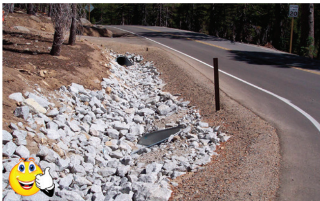
Good rock liner protection on this roadside ditch.
