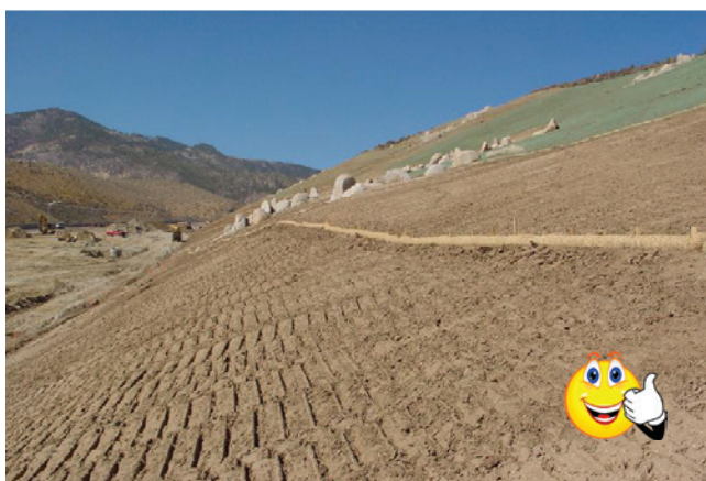
Great example of soil roughness - preparing for seeding
