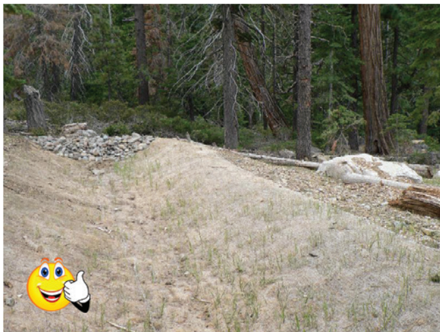
Vegetated water bar with rock cobble outfall
