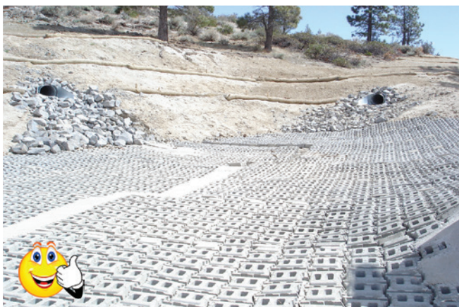
Excellent slope protection of highly erodible soils with fiber rolls, seed and hydromulch. Very good outlet protection and lining of a sediment retention basin with articulated concrete blocks.
