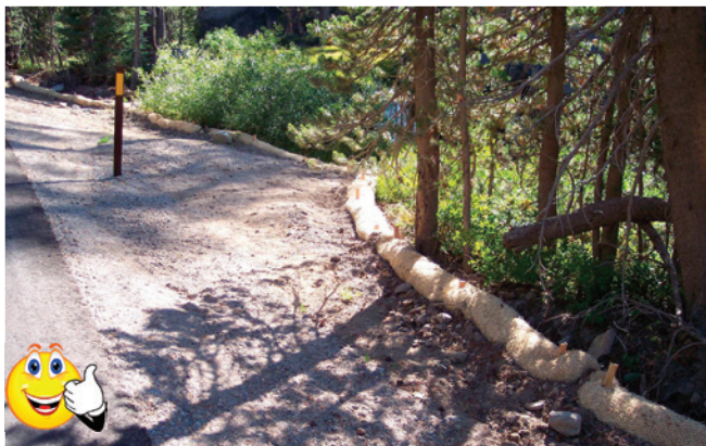
Good protection of a waterway located next to a road construction project with fiber rolls and a vegetated buffer. Fiber rolls must be overlapped by ~12" to prevent concentrated flows.
