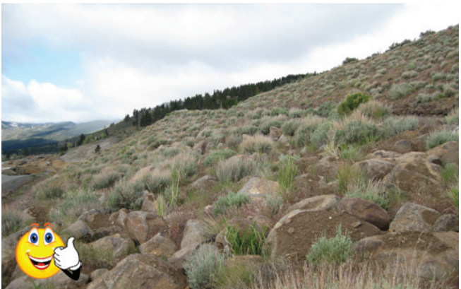
Rock riprap with salvaged topsopil and revegetation.
