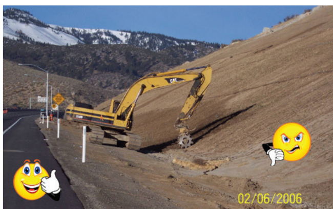
Great example of soil roughness - preparing for seeding
