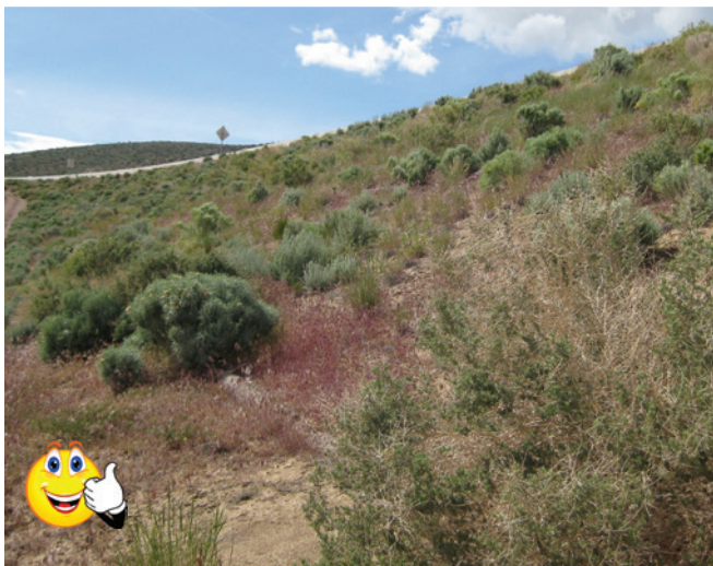
Good re-establishment of native vegetation on a long fill slope 2 years after seed applied.
