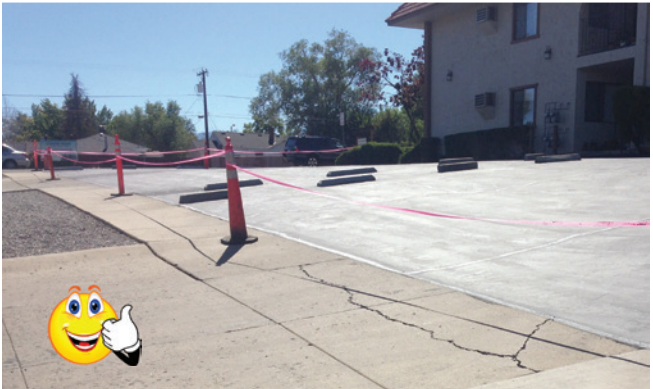
Excellent paving with no offsite contamination.
