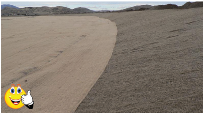
Excellent soil coverage at stream bank stabilization project using native seed and two types of biodegradable erosion control blankets.
