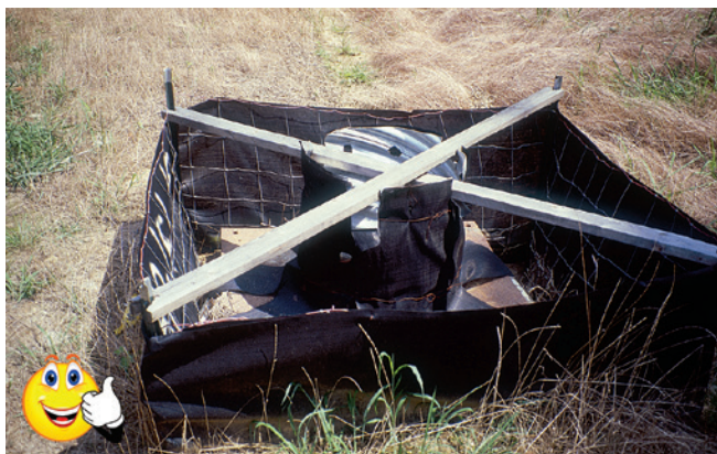
Good use of wire-reinforced silt fence to protect a low flow inlet. Note the diagonal bracing to protect against incoming flow pressures.
