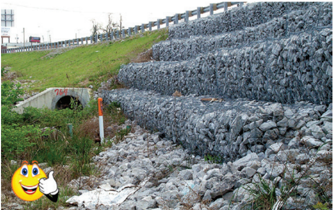
Good use of rock-filled stacked gabion baskets to protect steep slope. Soil and bark mulch can be used in or over gabions and planted with live willow or cottonwood cuttings to reduce the "hardened" look of gabions.
