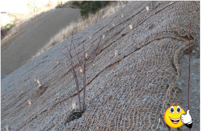
Great use of erosion control blanket with dowel anchoring system.
