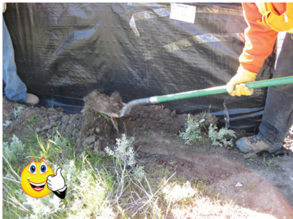
Correct installation method for silt fence. Key in and backfill.
