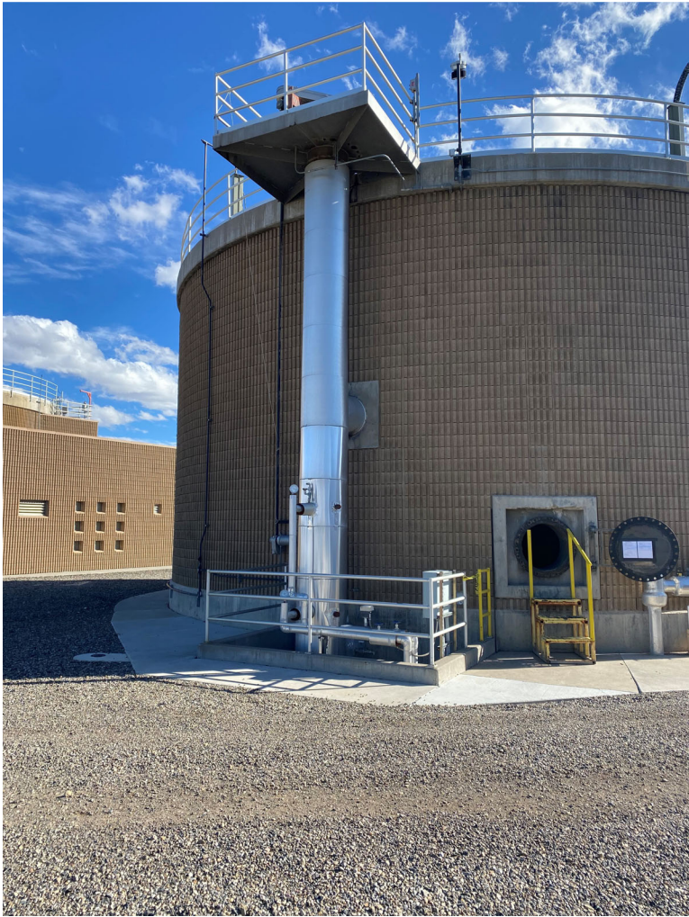
WEST SIDE MIXER TUBE ASSEMBLY
