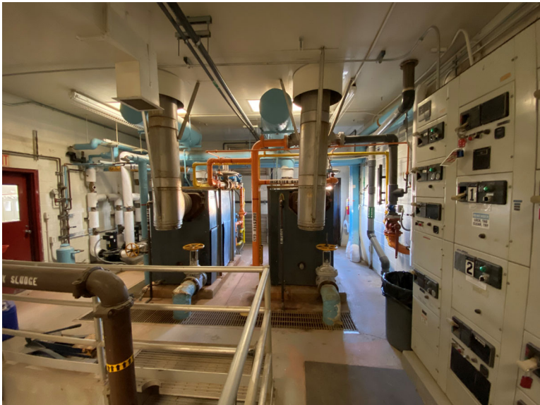
BOILER ROOM WITH TWO BOILERS TO BE REMOVED
