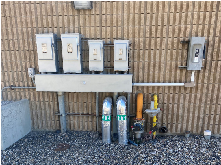
HOT WATER PIPELINES ENTERING/EXITING BOILER BUILDING
