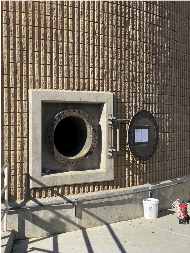
WEST SIDE ACCESS PORT DOOR ASSEMBLY
