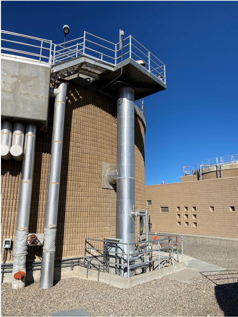
EAST SIDE MIXER TUBE ASSEMBLY
