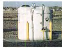
12. East Secondary Clarifier Hypo Tank
