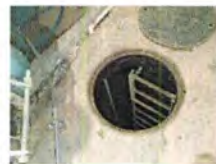
18. Effluent Wet Well
