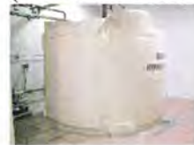
44. Plant Hypo Tanks (North and South)
