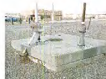
30. Head Gate Valve Vault
