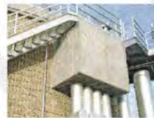
74. Secondary Digester Overflow Box
