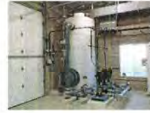
36. Headworks Potable Water Tank
