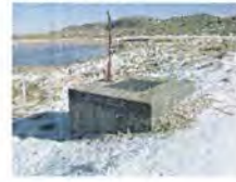
58. RIB 1A and 1B Distribution Valve Vault
