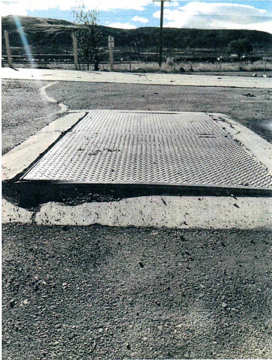
5180 Idaho St. – Deteriorated Vault.
