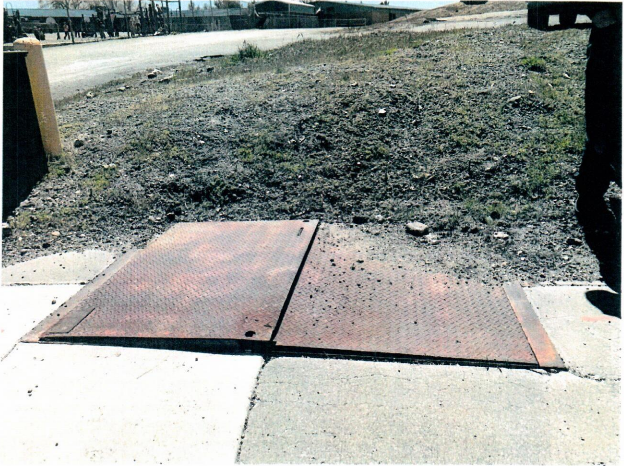
Sewell Drive Vault – Damaged Vault lid.
