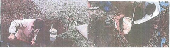
Final hand digging up of spaces in RV park that broke due to excessive water pressure and blew lines. This is after 4 feet of digging with excavator.
