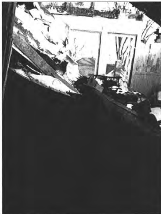
PHOTO 34 - BEDROOM (NORTH SIDE) 2ND FLOOR - COLLAPSED ROOF
