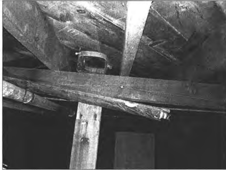
PHOTO 13 - TYPICAL POST & BEAM BENEATH MAIN FLOOR
