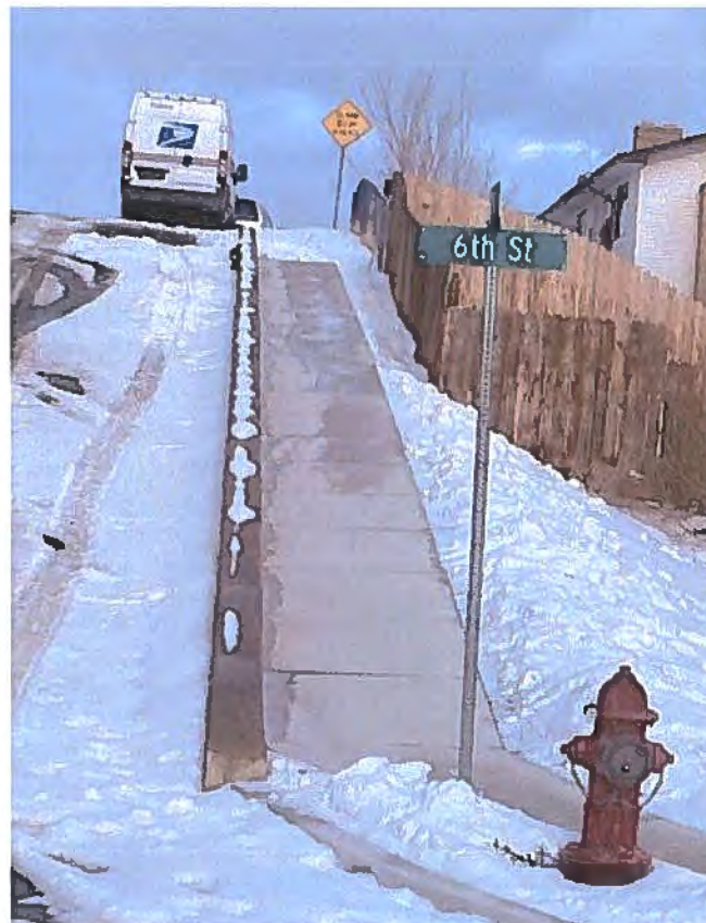
Exhibit D – Sidewalk with Retaining Wall (W Cedar/D St.)
