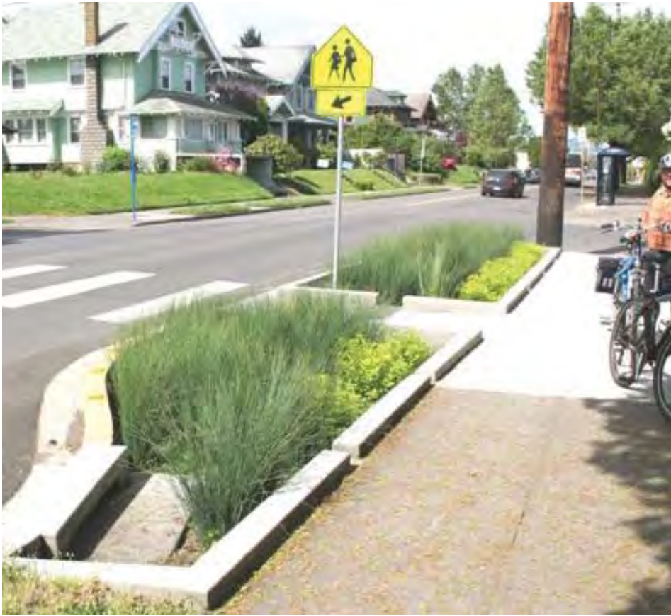
Roadside rain gardens are swale-like planted areas to mitigate stormwater runoff.
