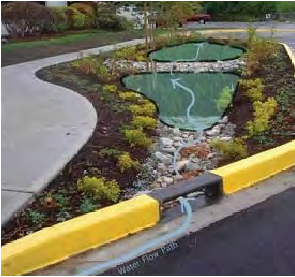
This bioswale area on the curb collects water in gravel/stone-filled channels on surface, filtering into the ground.
