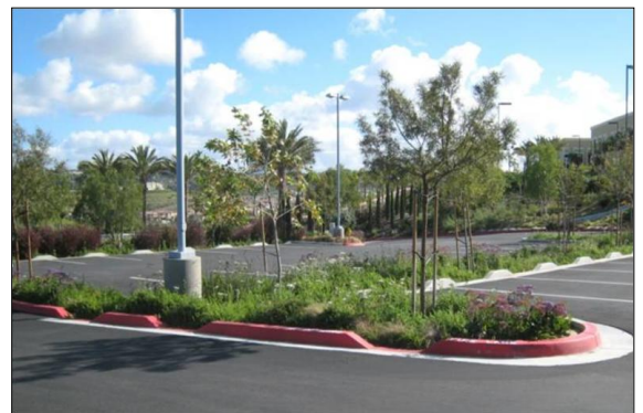
Illustrative example of a continuous planting strip between planter islands and breaks in the curb to allow stormwater to enter.
