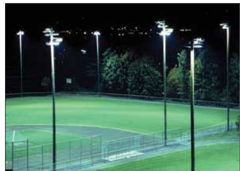
Illustrative example of lighting that cuts off candlepower above the horizontal level by using "full cutoff luminaires."
