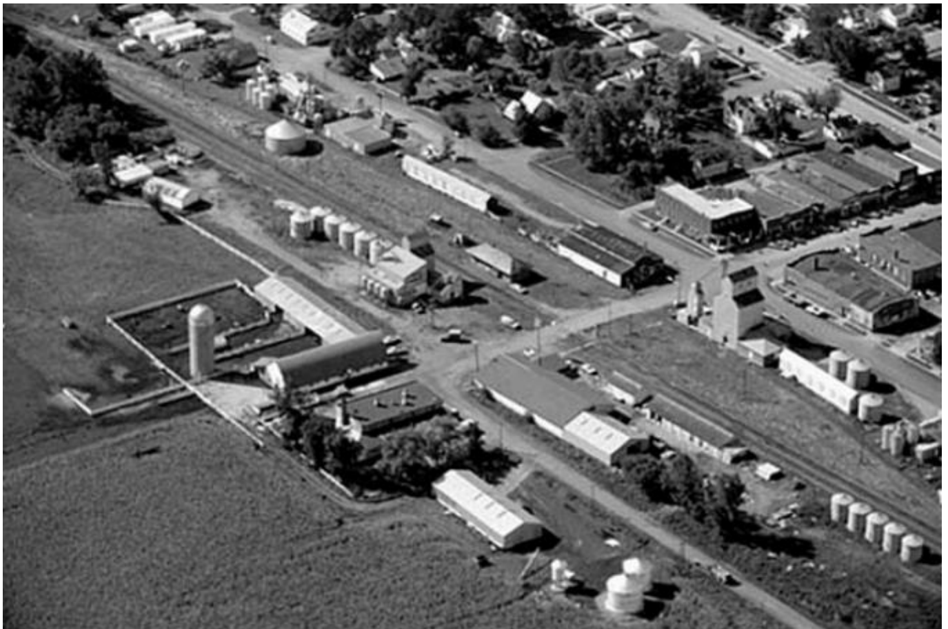
Elevator and surrounding area, 1972
