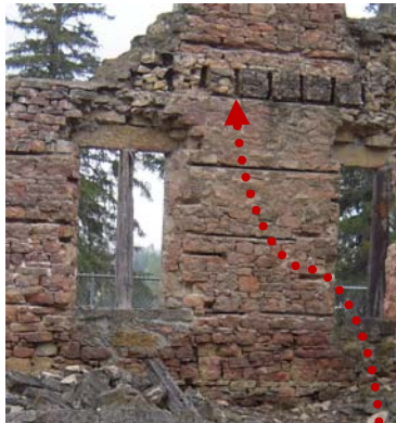
Joist pocket once held the second floor joists
