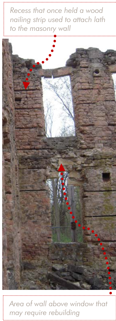
Interior face of wall (5/20/2014)
