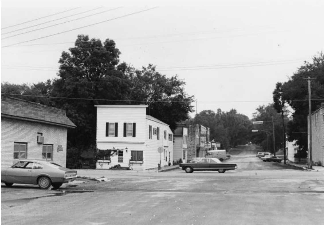
Mantorville Historic District, 1972.
