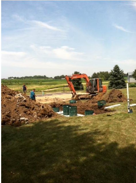
Installation of a new septic system in rural Dodge County.
