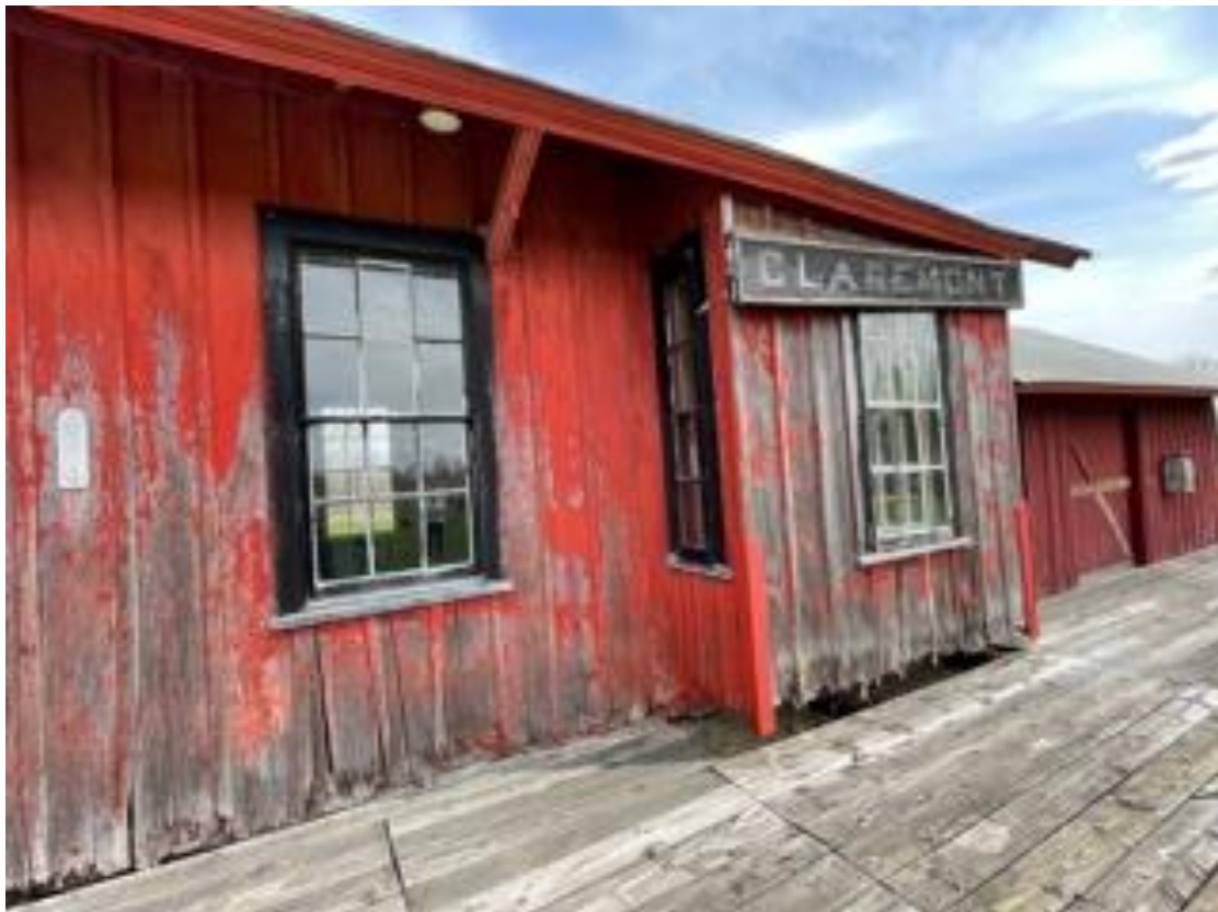
Old Claremont Train Depot (front)
