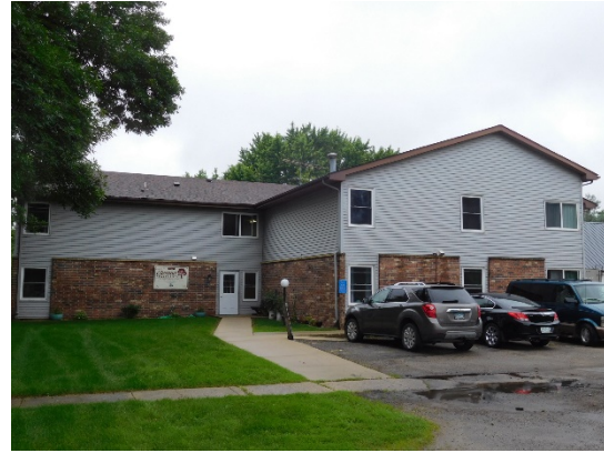
Subsidized GO Rental in Mantorville
