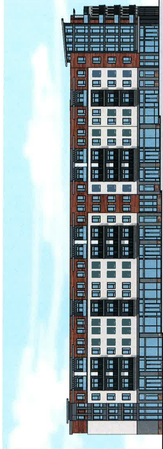
APT BUILDING #1: LOOKING SOUTHWEST
