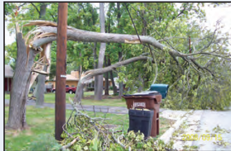
Tree on utility lines on Kenwood Road. Thousands were without power for multiple days due to tree & wind damage.
