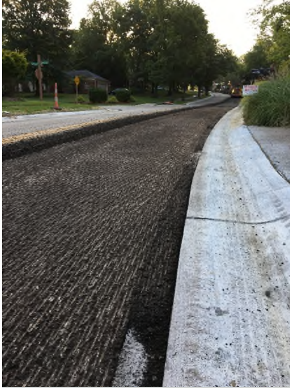
Milling of Old Roadway
