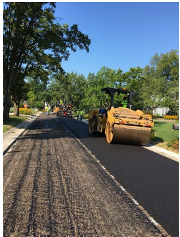
Paving New Road Surface
