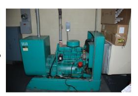
**Description:** This project is to replace an existing generator that provides power to the fire/rescue building. The current generator was installed in 1979.
