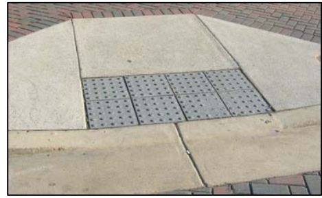
Image of installed detectable truncated domes at the end of a curb ramp
