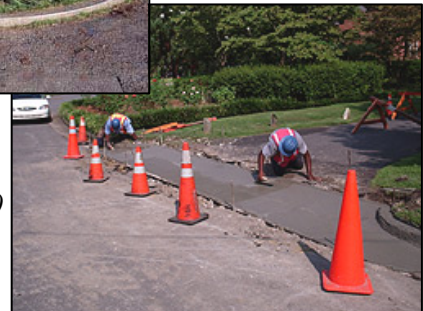
Images of sidewalk maintenance & retrofit Courtesy of Dan Burden ( www.pedbikeimages.org )
